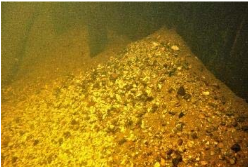
Figur 42: Utfallet stenmaterial genom glipor i spont.
